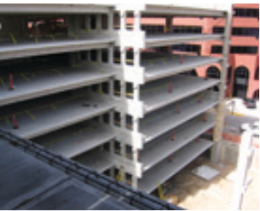
Structure included pretopped double tees, litewalls and thin brick panels.
