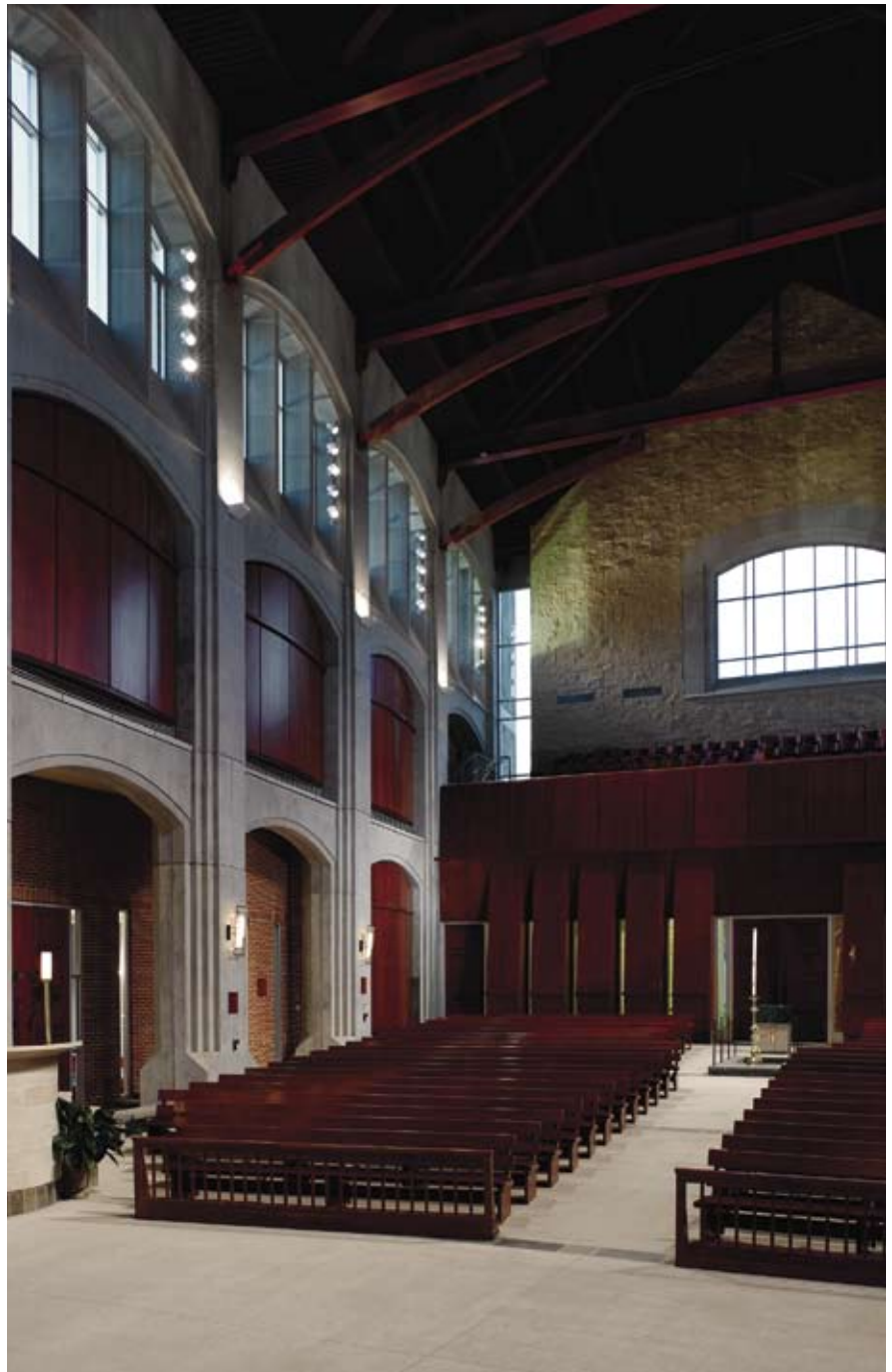
Fig. 5. Precast concrete arches emulate the traditional architecture of historic worship spaces and simultaneously create the modern aesthetic of natural stone. (Courtesy of Brian Dressler)
